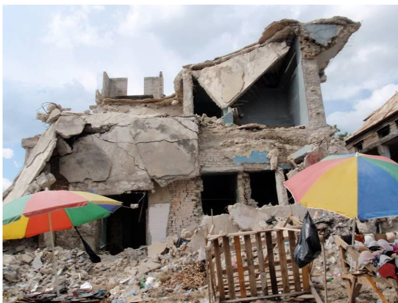
Building in down town Port au Prince
